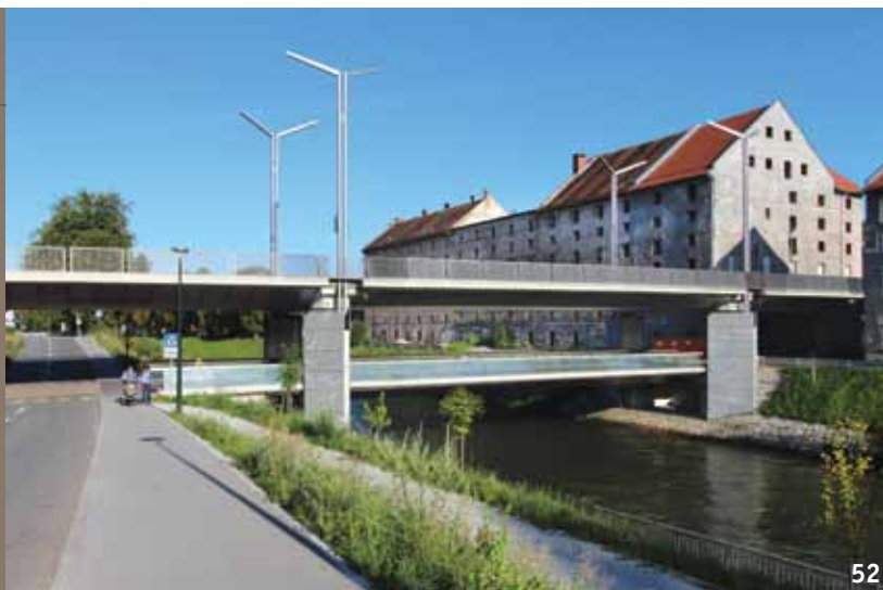
52 Fabianijev most čez Ljubljanico med Roško in Njogoševo cesto, 2012, arh. Jurij Kobe Fabiani Bridge across the Ljubljanica River between Rog Street and Njogoš Street, 2012, Arch. Jurij Kobe
