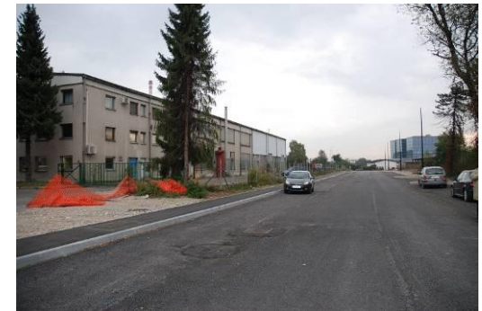
OBSTOJEČA HALA, KI SE OHRANI
